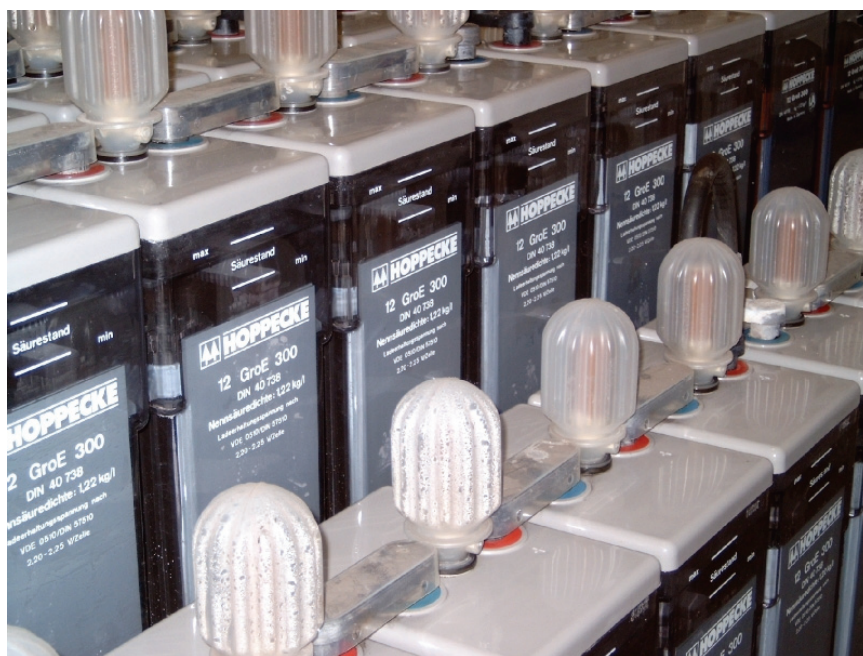
Fig. 9 – With proper design the catalysts can reach an age of more than 20 years (units installed in 1984)
