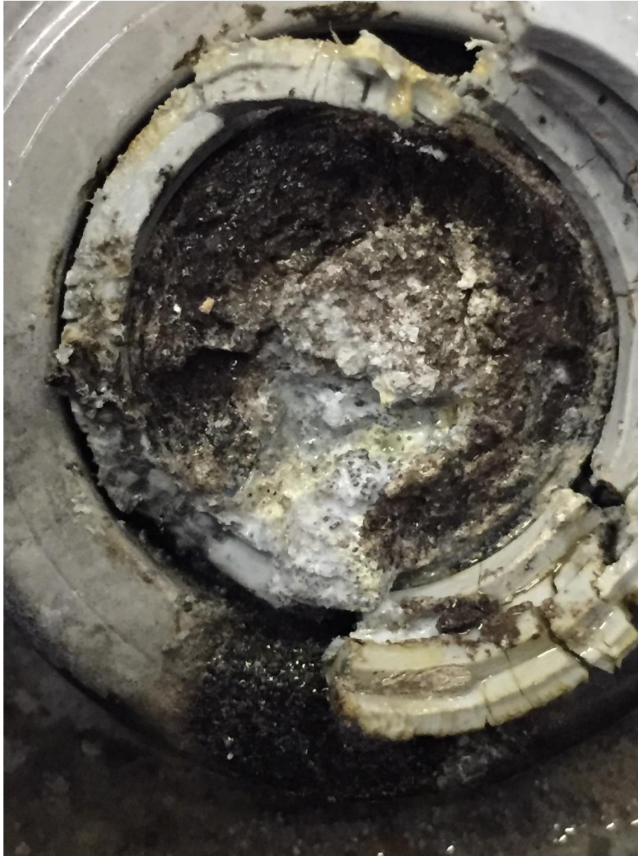
Figure 23 is a closeup of the upper portion of the post from the previous picture. This is within the post seal well. As can be seen the metallic structure has undergone severe change. This post melted open but the cell did not explode.
