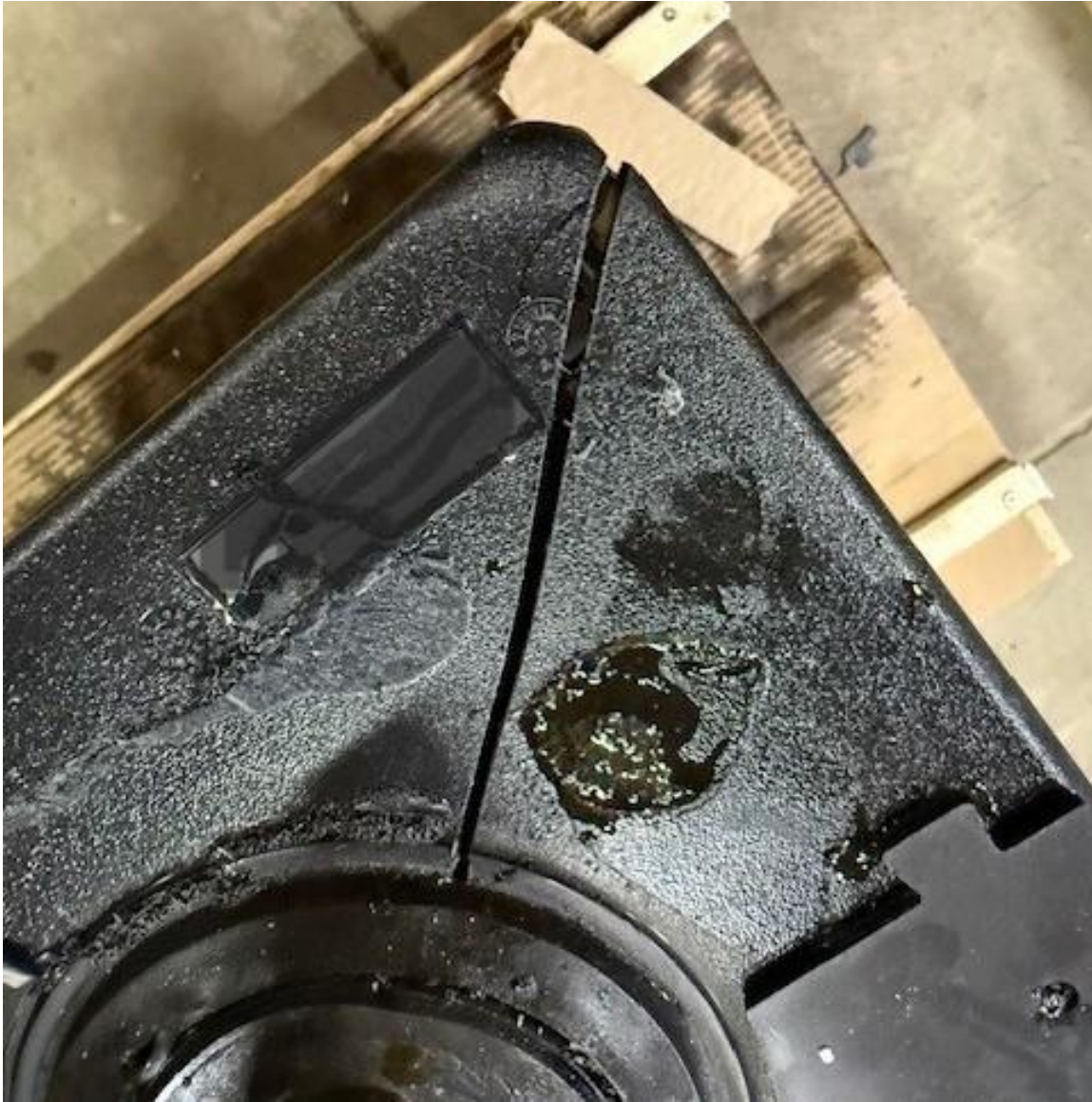
Figure 33 shows a cover with an extremely well-advanced crack that has turned at the edge of the cover and started down the side of the jar. This cell is over 19 years old.
